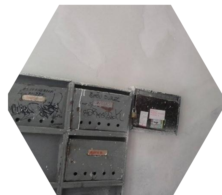
Apartment building renovation in Budisov
